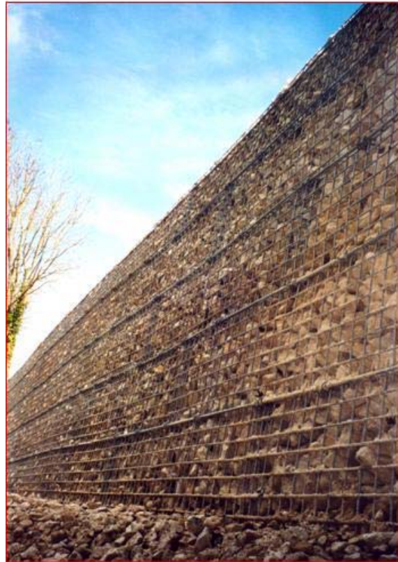
Figure 11: Slope reinforcement on the secondary road 514 in the "Moulin de la maison Fort" in Bitry – Nièvre- France
